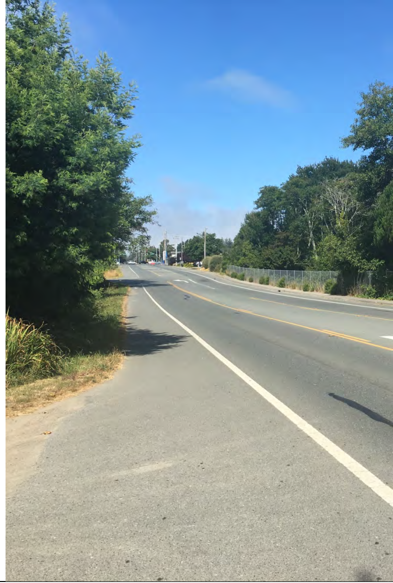
SOUTH SIDE OF ROADWAY 2020-07-17 EASTBOUND
