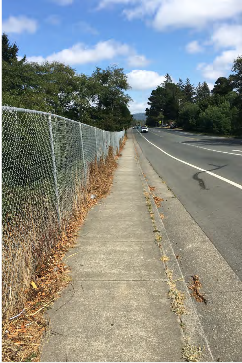
NORTH SIDE OF ROADWAY 2020-09-04 WESTBOUND
